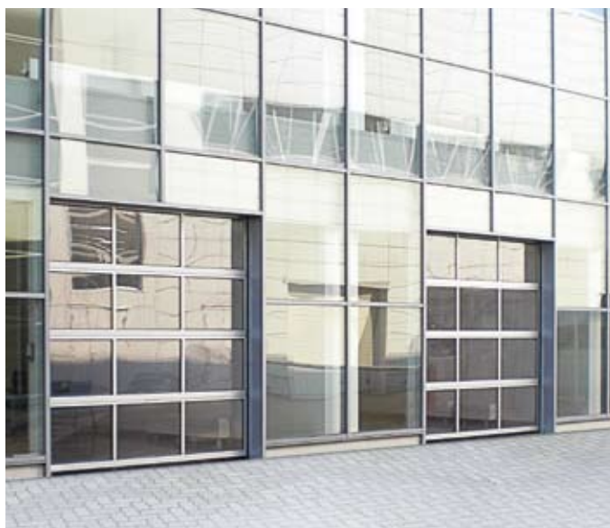
Glazed panoramic panels of aluminium profiles form a door leaf
